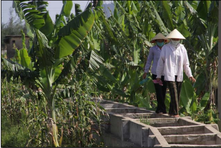
A new canal built to provide fresh water for saline fields.
